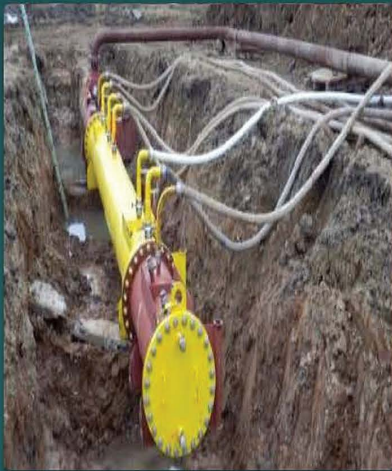
Before the hydro test 1- water filling
